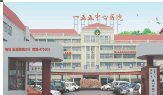
The 155th Central Hospital of the people's Liberation Army in Zhengzhou, Henan Province Direct drinking water supply system project
