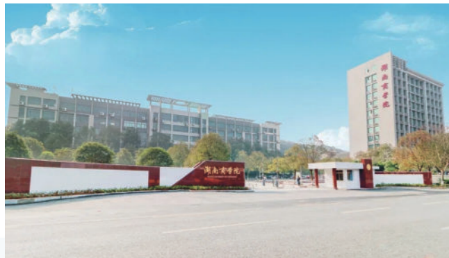
Hunan Changsha business college Direct drinking water supply system project
