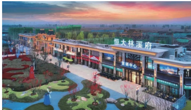
Anhui Fuyang Hengda Linxi Direct drinking water supply system project
