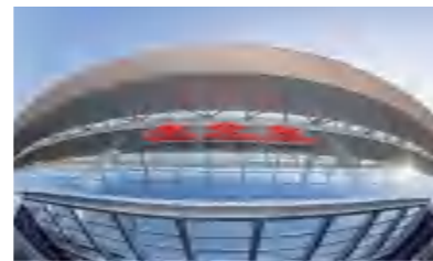
中铁十二局集团京雄城际铁路雄安站 Beijing Xiongan Intercity Railway Station of China Railway 12th Bureau Group
