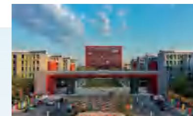
庐江新二中 Lujiang New No.2 Middle School
